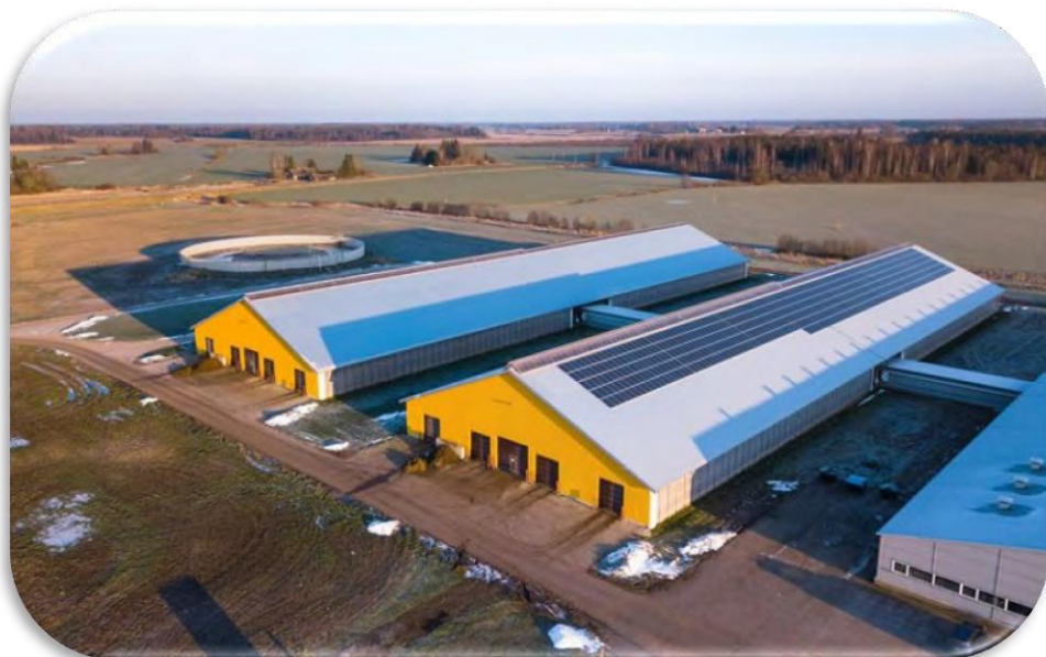
1.1MW Solar Power Plant Estonia year 2019
