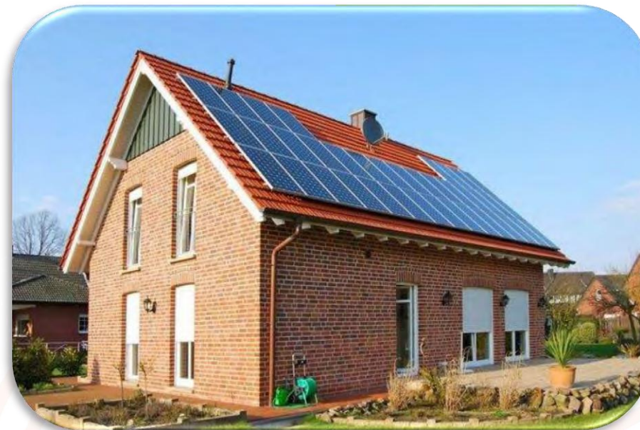
500kw Roof System Germany year 2014
