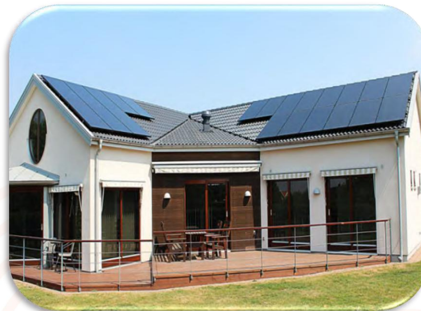
300KW Residential Roof Solar Power Sweden year 2016
