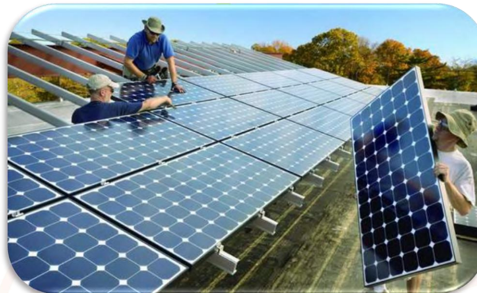
800kw Power Plant Chile year 2016
