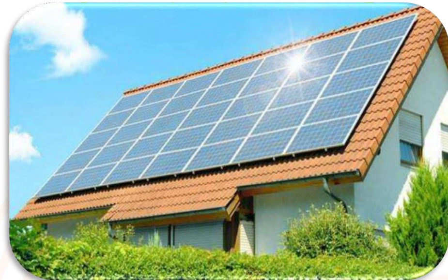
800kw Roof System Netherlands year 2014
