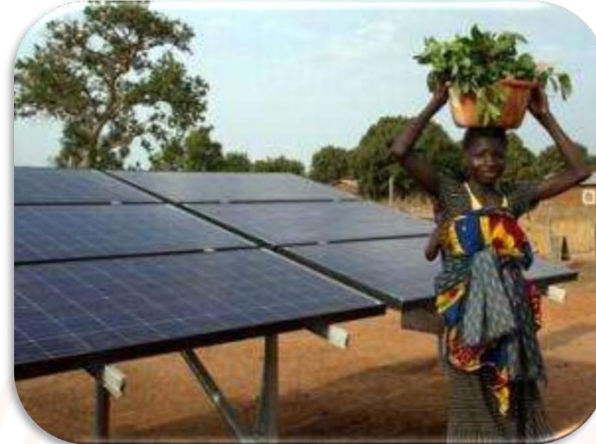
200kw Solar System Nigeria year 2018
