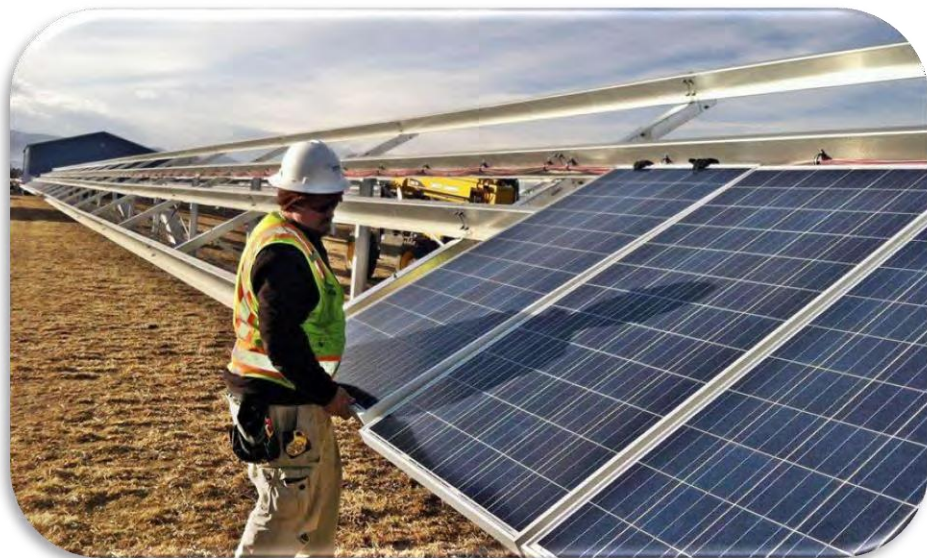
3MW Power Plant Belgium year 2014
