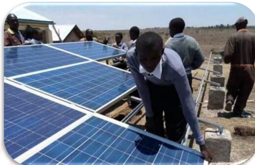
800kw Solar System Angola year 2018
