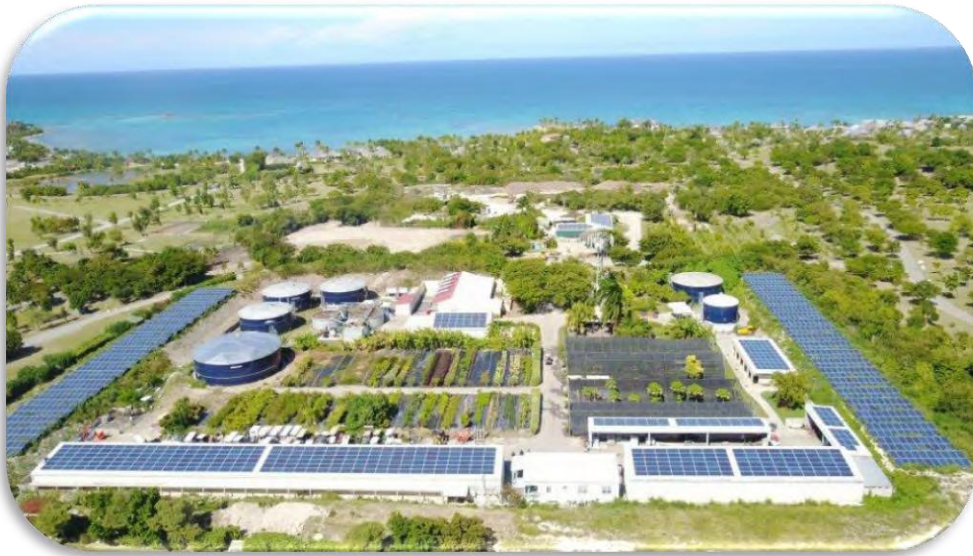
404kw Solar System Jumby Bay year 2017
