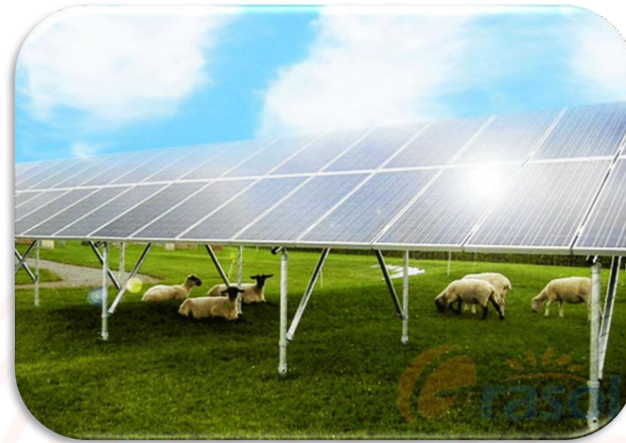
1MW Power Plant Switzerland year 2016
